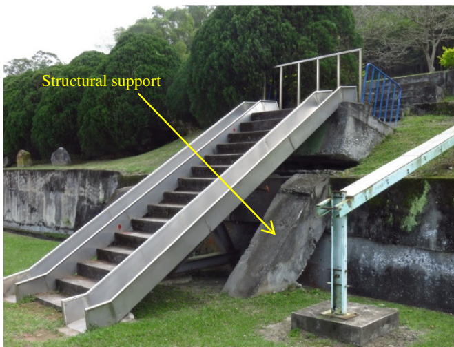
Figure 15. Structural supports of retaining wall against horizontal movements at Dapo Elementary School
